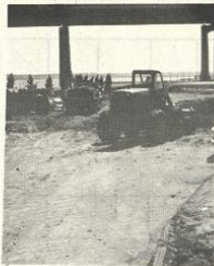
The new tennis courts take shape
