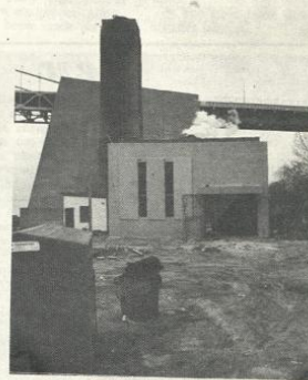
More power to the powerhouse.
